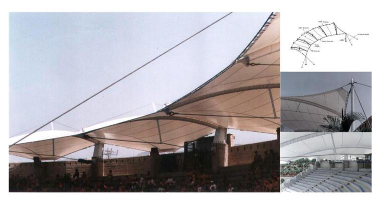
The roof built over the existing stands of the dolphinarium in Tenerife has a covered surface area of 2,300m2 with a 15.0m overhang. The main condition required for the project was to build the roof without interrupting the day-to-day functioning of the Park.
